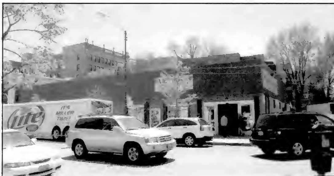
Non-contributing building at 1031 West Argyle Street
